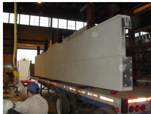
Figure 1.4- Prefab Section on Truck
