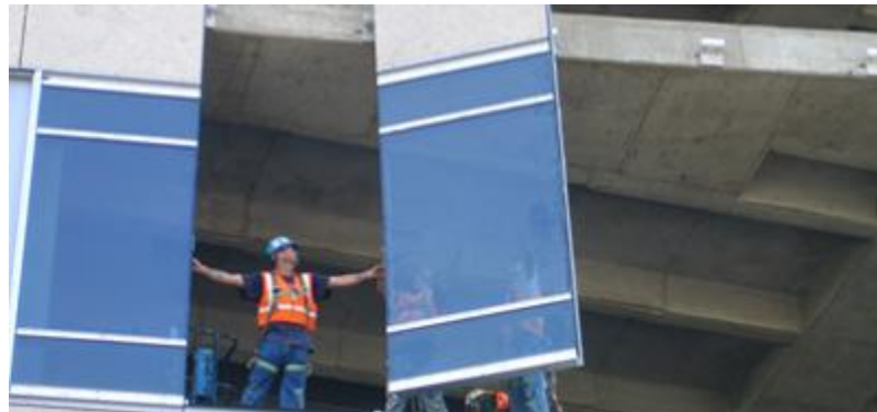
Figure 1.2 Placing a Prefab Curtainwall Section on a Similar Building
