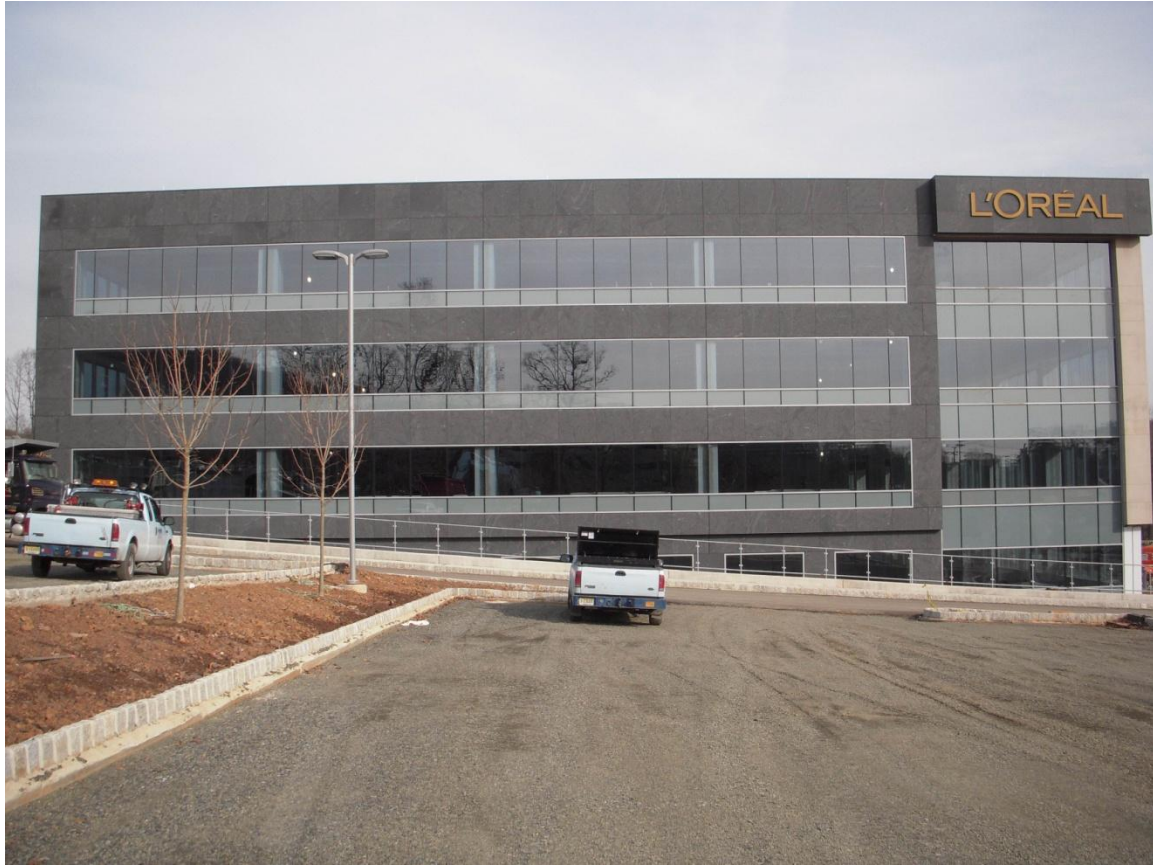
Figure 1.3 - Finished West Facade
