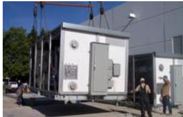
Figure 3.8 Placing equipment on grade
