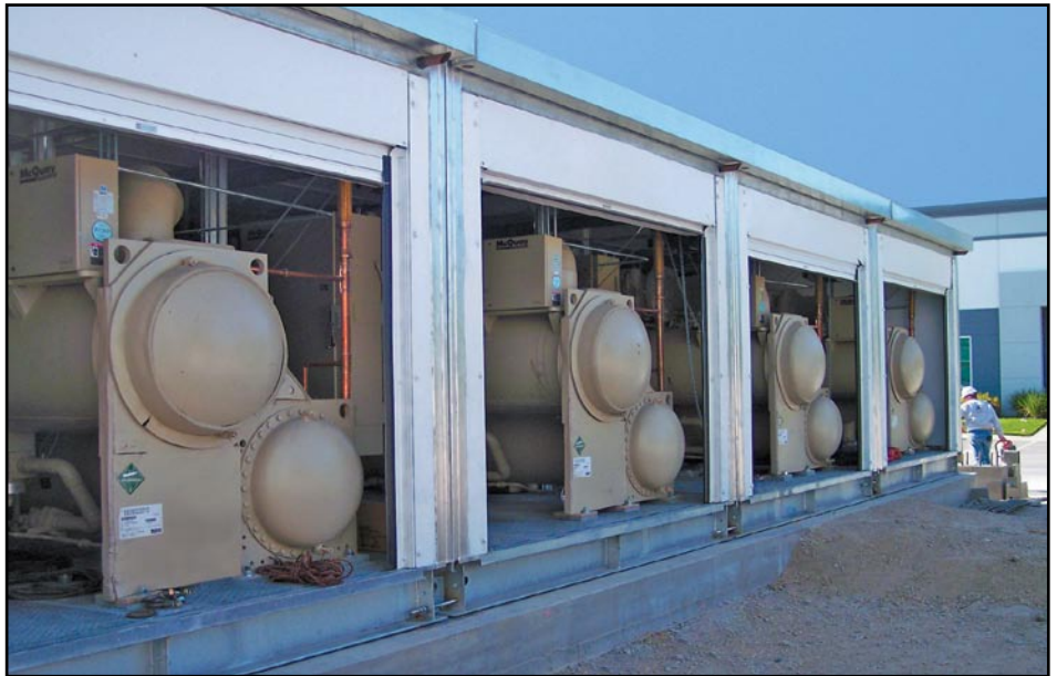
Four of the six McQuay Modular Central Plants that provide mission critical cooling for the Herakles Data Center.
